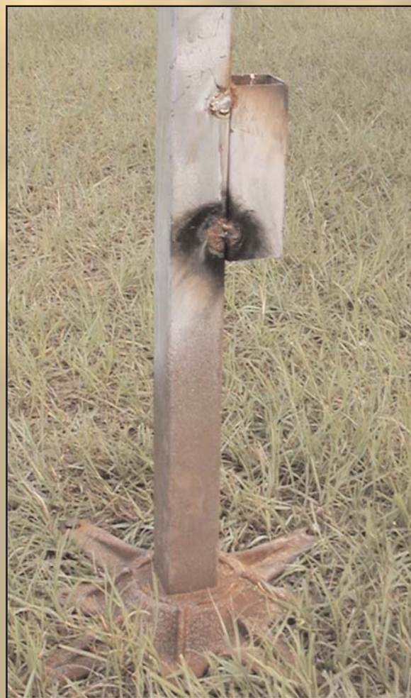
Close up of wall stand showing welded on 2 ½" channel. The channel allows for a series of panels to be placed in line or to establish a right angle for a hallway or room.
